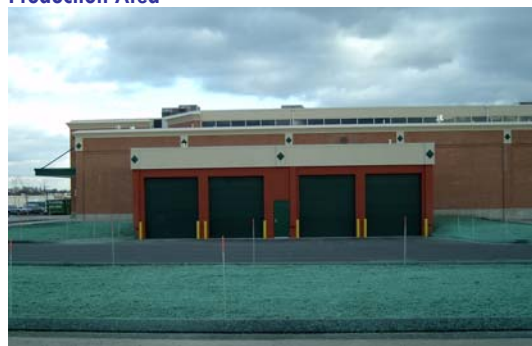
New Loading Dock
