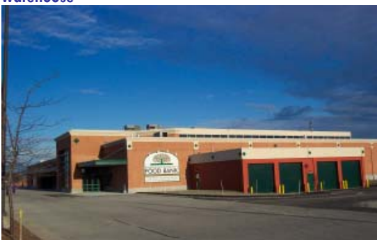
Front Entrance and Loading Dock
