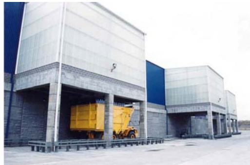
New Loading Bays
