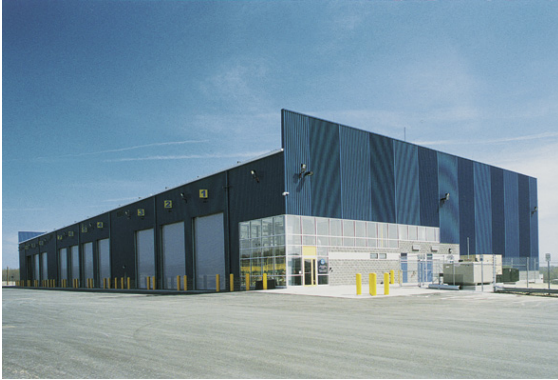
New Tipping Facility
